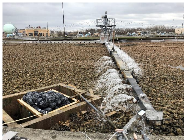
Figure 1: Trickling filter with test bed pictured with four rotating arms and water flowing over rock media.
